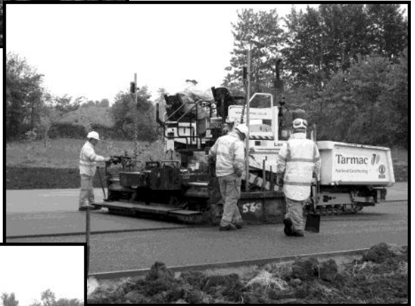
Levelling the tarmac
