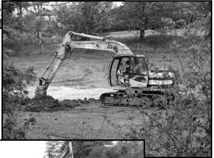
Levelling the soil in the base area
