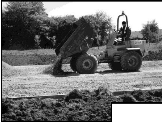
Laying the hardcore
