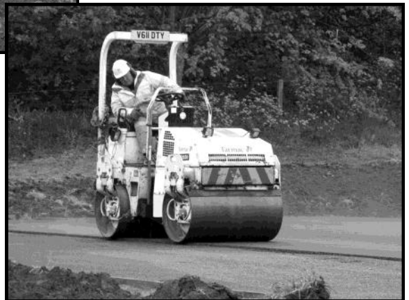
Rolling and compressing the finished surface
