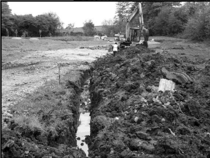
Draining the site
